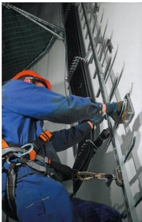
Height access system with fall-arrest device at a fixed guidance EN 353-1.
